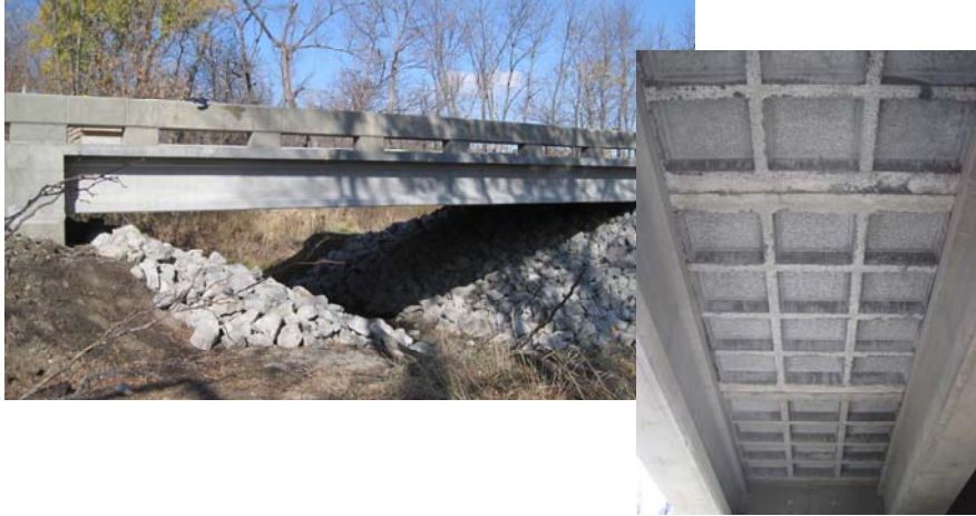
Dahlonge Road Bridge in Wapello County, Iowa
