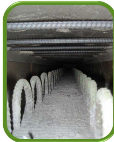
Concrete Girder Connection
