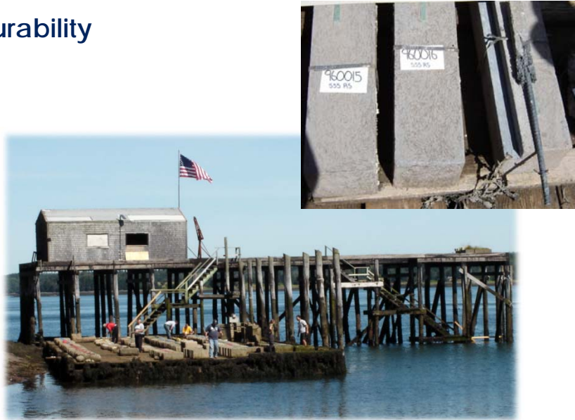
USACE Facility at Treat Island
