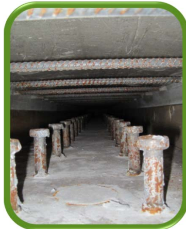
Steel Girder Connection
